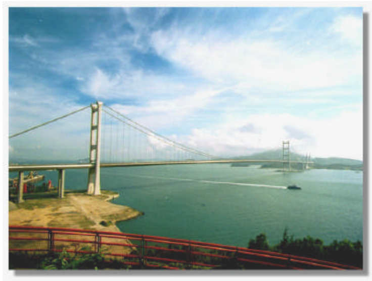
Tsing Ma Bridge
