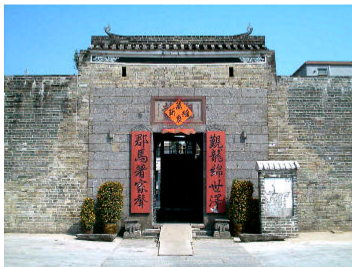
Gate Tower of Kung Lung Wai
